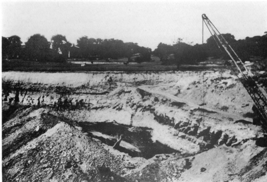
Fig. 2. General view of the north east corner of the Catstone Hill opencast coal site, looking down onto the Dunsil Coal.
